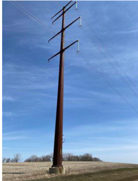
Figure 6. Double Circuit Structure
